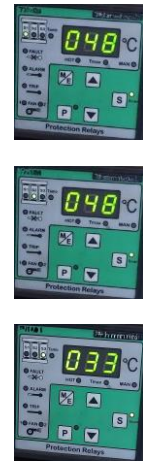
Fig. 4. The S3 channel temperature sensor was replaced on 19/05/2022. 406kWp photovoltaic plant. The ambient temperature on the same date and time was 12.5°C (at the weather station installed near the substation).
