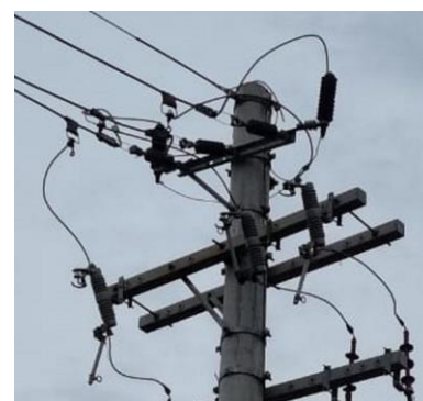
Fig. 11. On 02/05/2023, the main switch installed in the 444kWp photovoltaic plant caused a short circuit followed by a fire in the plant's substation. One of the fuse links did not break, leaving the three-phase circuit energized after the incident.
