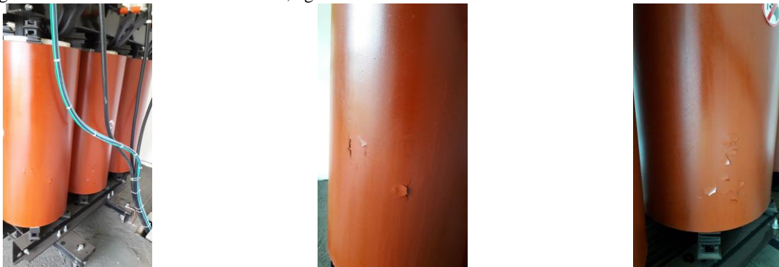
Fig. 1. The transformer installed in the substation of the 406kWp photovoltaic plant. As of the date of the image, 04/12/2021, it had not been energized, but already showed degradation of the fiberglass insulation.
