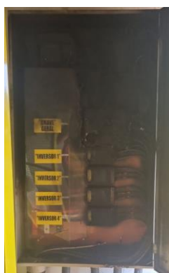
Fig. 11. On 02/05/2023, the main switch installed in the 444kWp photovoltaic plant caused a short circuit followed by a fire in the plant's substation. One of the fuse links did not break, leaving the three-phase circuit energized after the incident.
