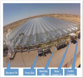
Figure 16: Detailed layout of the Miraah structure in Amal
