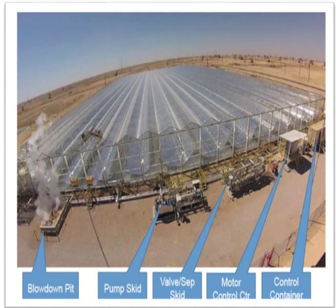
Figure 16: Detailed layout of the Miraah structure in Amal
